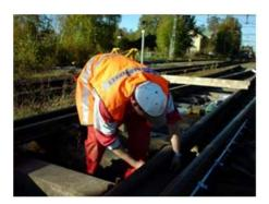
In some extreme cases where the switch is in an exposed position with heavy winds or where large amounts of snow can be expected, an extra element is mounted on the moving rail. This element is mounted on the side facing the stock-rail.
