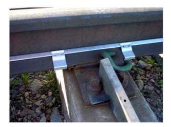
Fit the next channel tightly against the first one, and it is a good idea to make a clip cover the joint.
